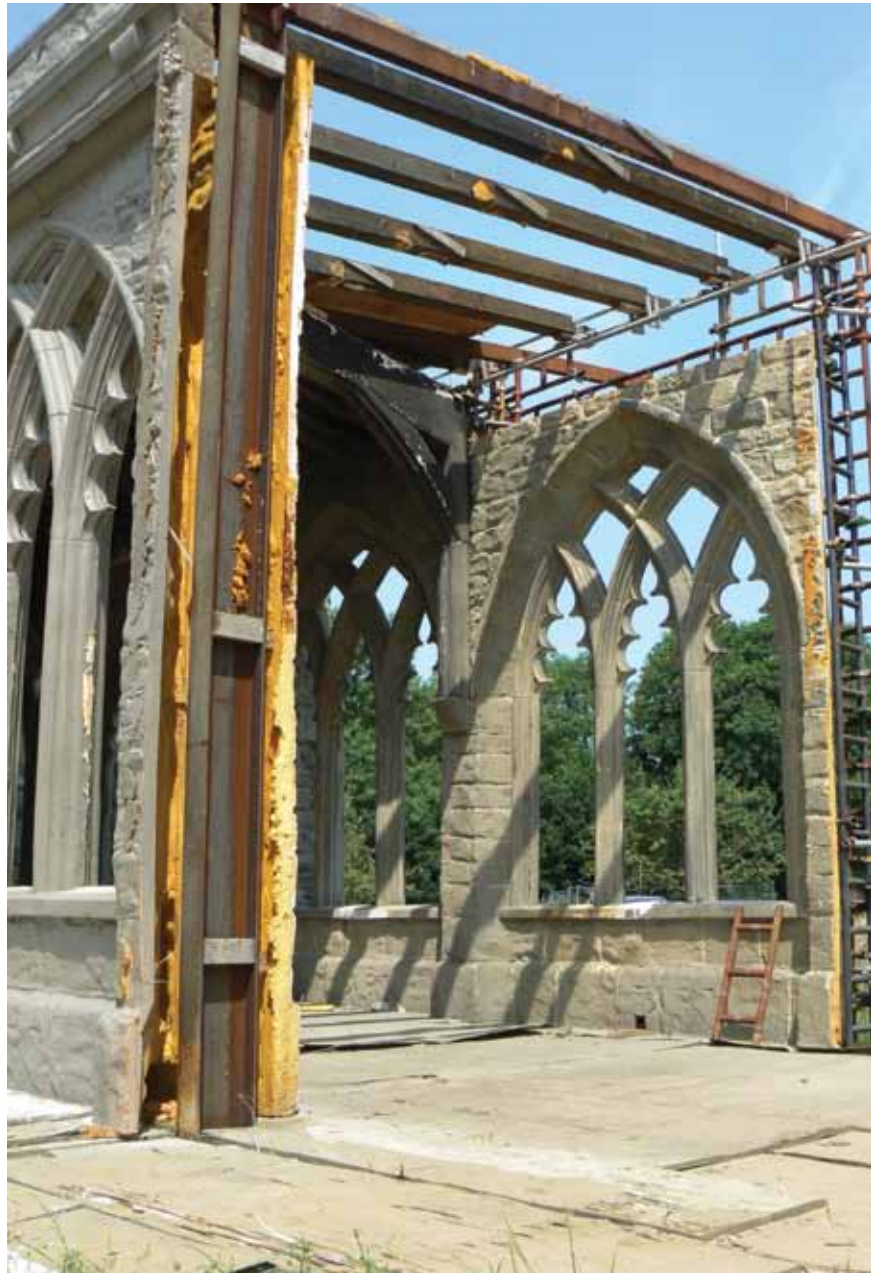
Opposite page: Stuart Craig's original pencil drawing of the memory cabinet for Headmaster Dumbledore's office. Inset: A photograph of the finished prop. Above: A piece of the exterior of Hogwarts' central courtyard set, revealing the polyurethane foam tracery panels.
