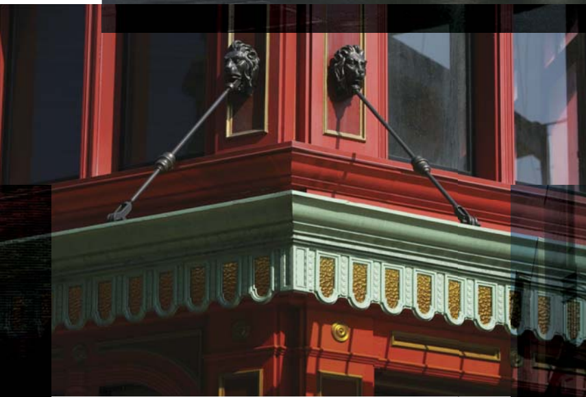
Above: This detail is from the corner of Block 12 at the west end of New York Street. Beala modified the design of the previous façade making it a story higher, and added the awning with the glass and stamped metal filigree and gold trim from the W.F. Norman Co. in Missouri. The staff work was executed in fiberglass and resin by Local 755 craftsmen from the Universal Studios staff shop. Right: The west side of Courthouse Square includes a firehouse with doors large enough to allow a pumper truck to drive in or out.
