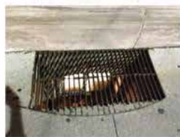
grate over window well
