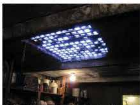
glass block skylight
