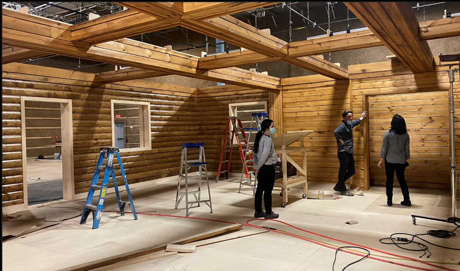
INT. DEERFIELD MOTEL LODGE BUILD PROGRESS PHOTOS
