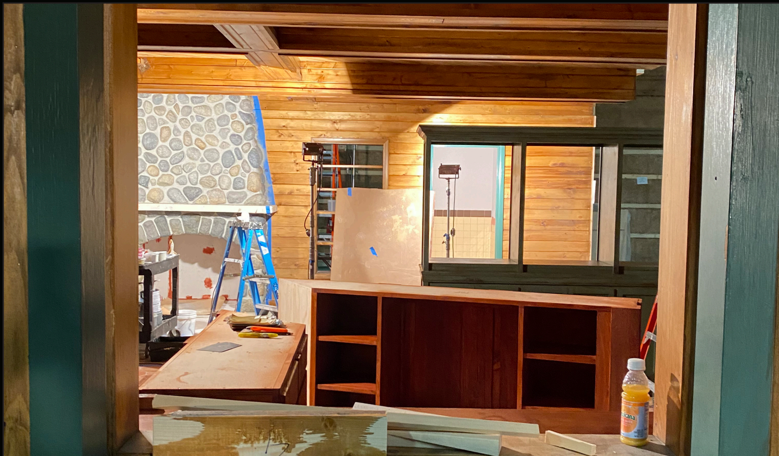
INT. DEERFIELD MOTEL LODGE BUILD PROGRESS PHOTOS
