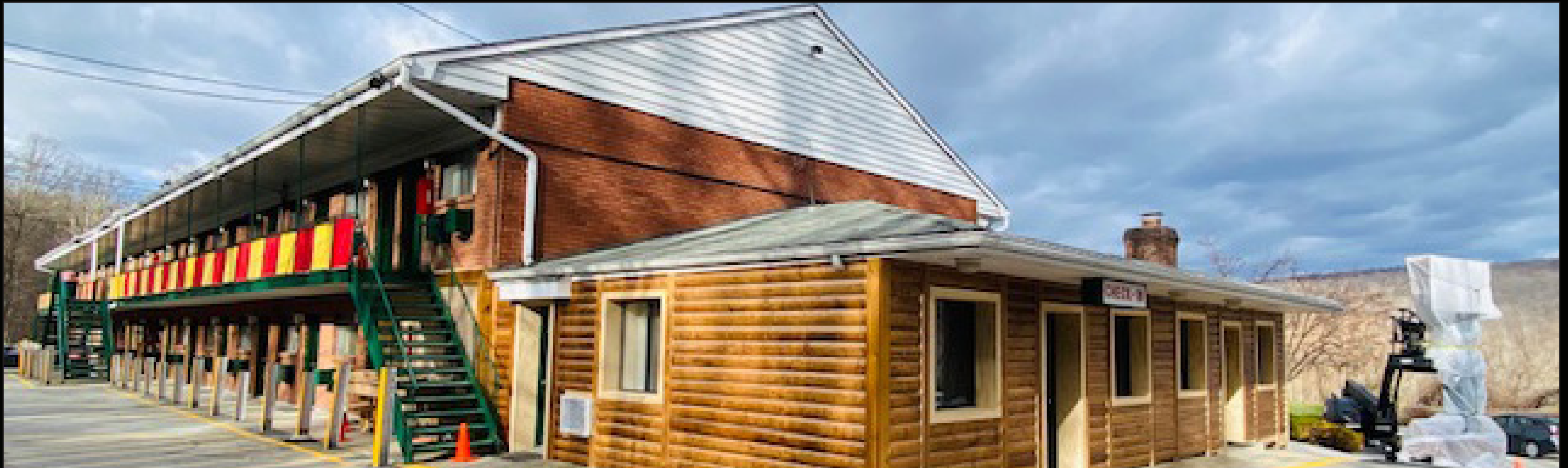
EXT. DEERFIELD MOTEL BUILD PROGRESS PHOTOS
