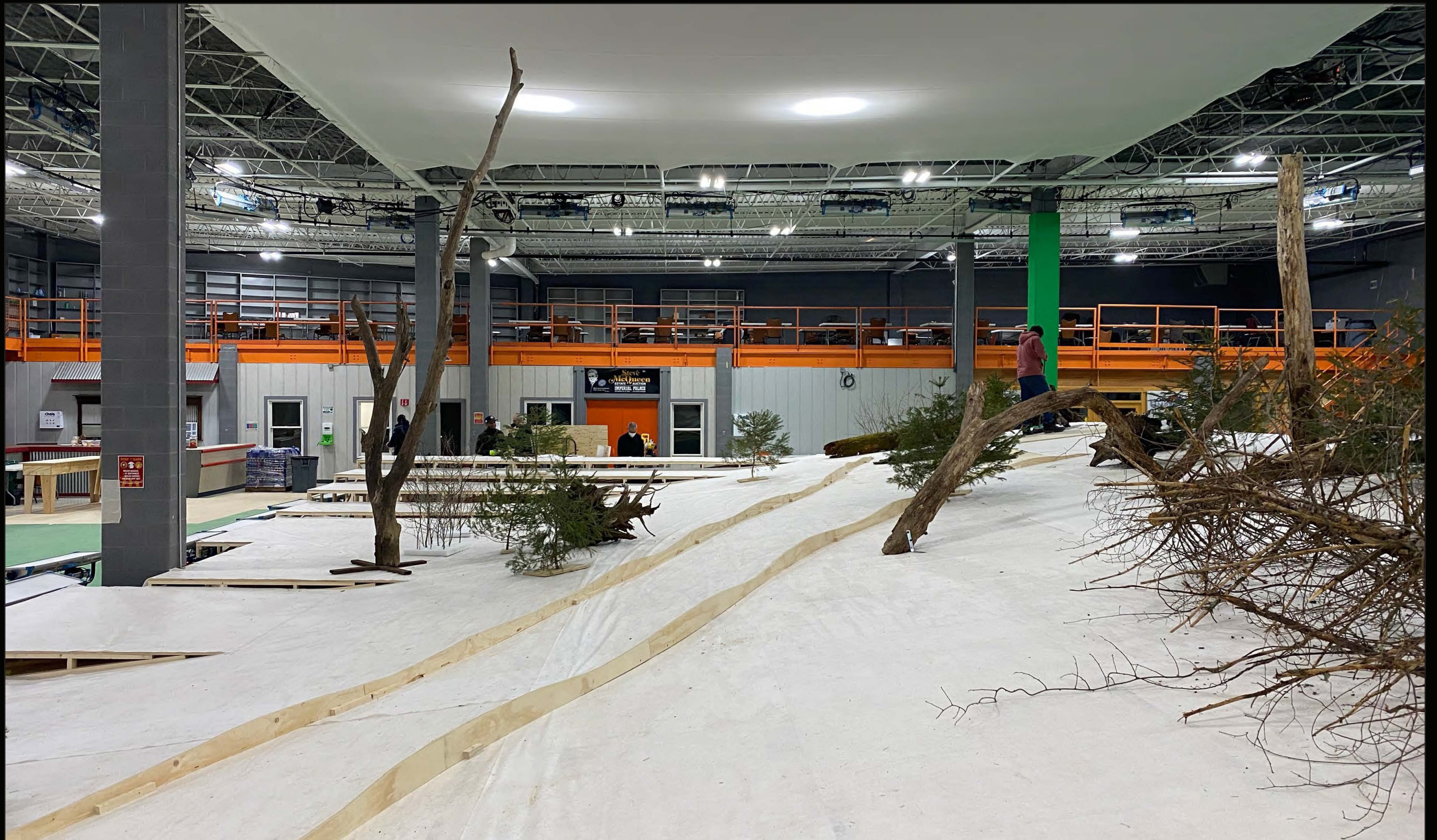
I/E "THE SPOT" - TREE HOLLOW STAGE BUILD IN PROGRESS
