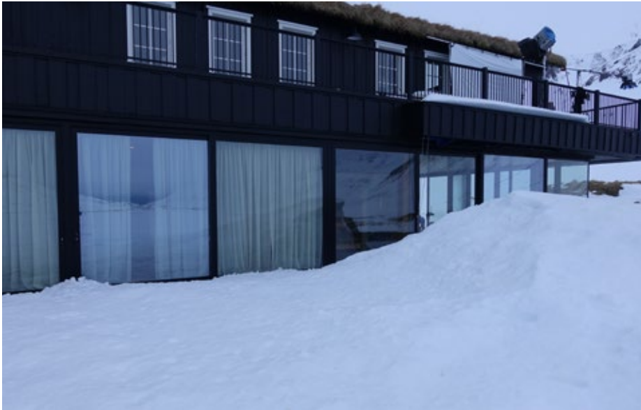
Deplar Farm – Location Photo
