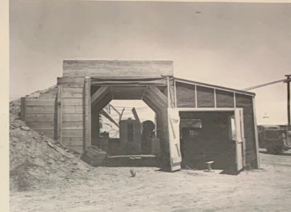
Power plant at B.
