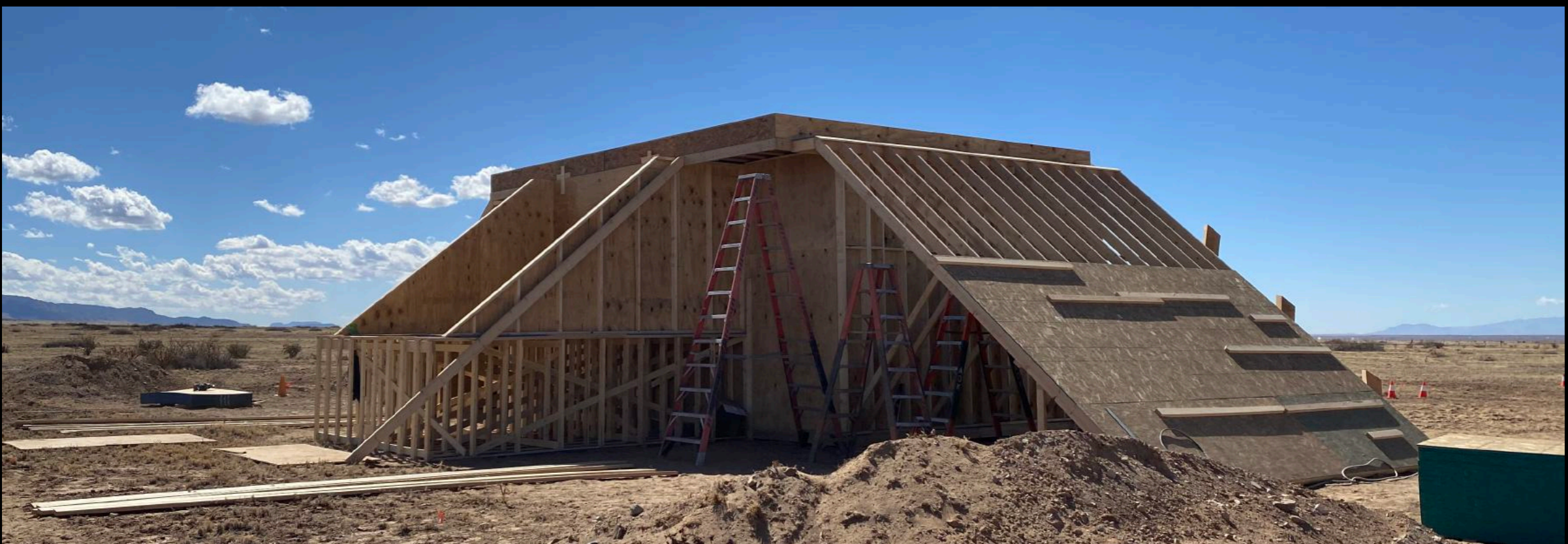
10,000 S Observation Bunker - Build
