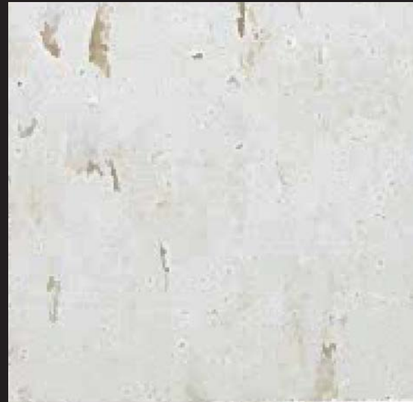
Hallway Floor Tiles
