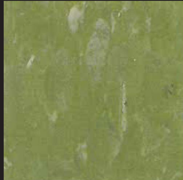
Hallway Border Floor Tiles
