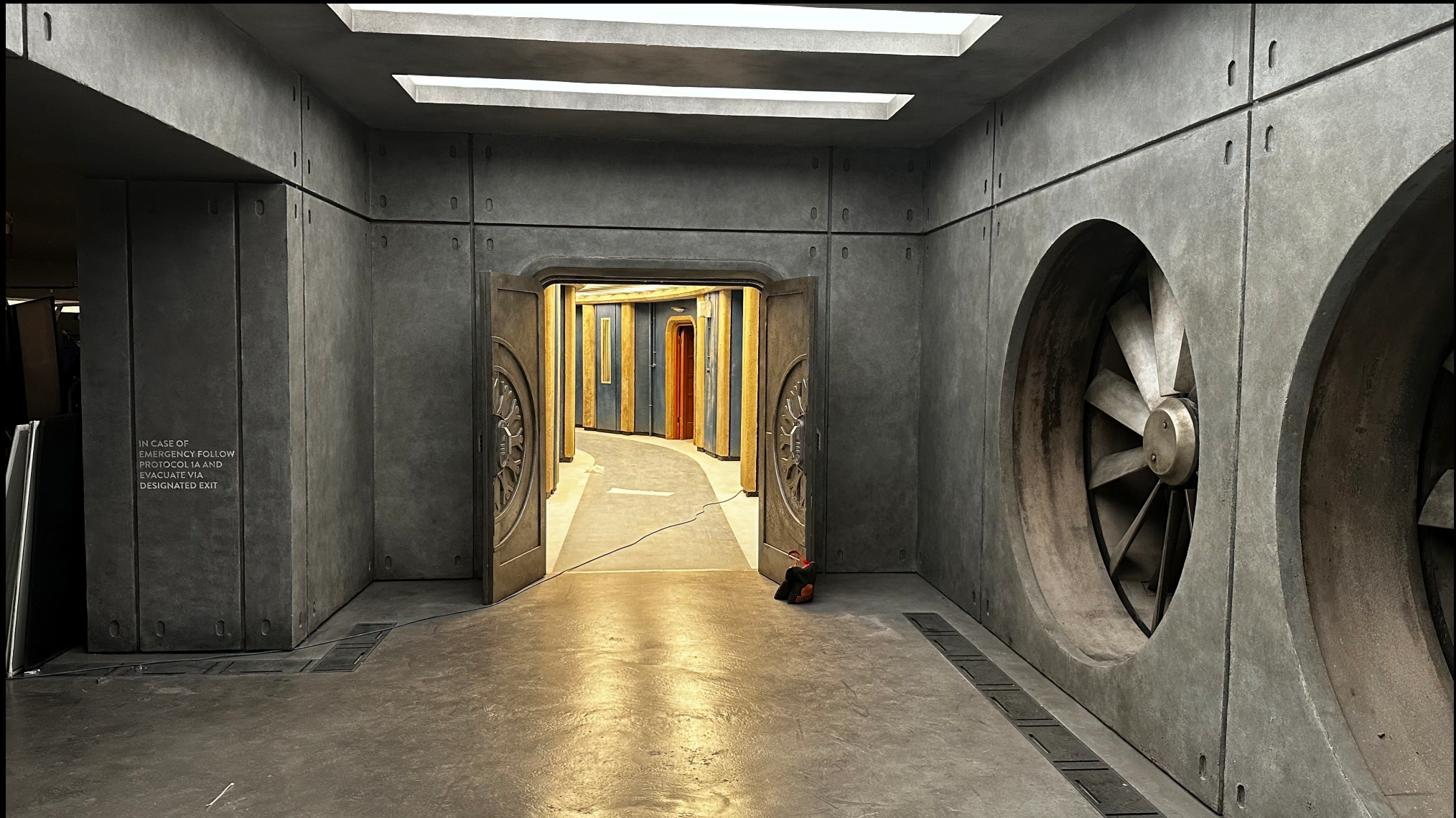
Silo 18 – IT Server room – Set
