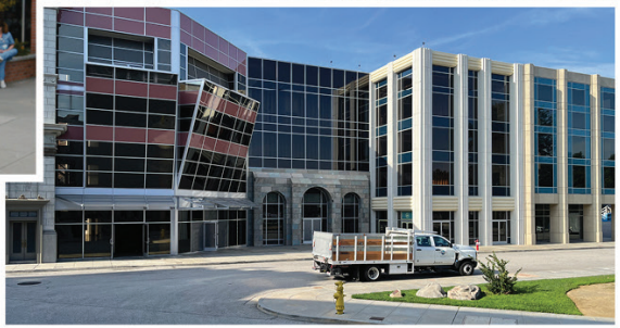
EXT. Before Facade
