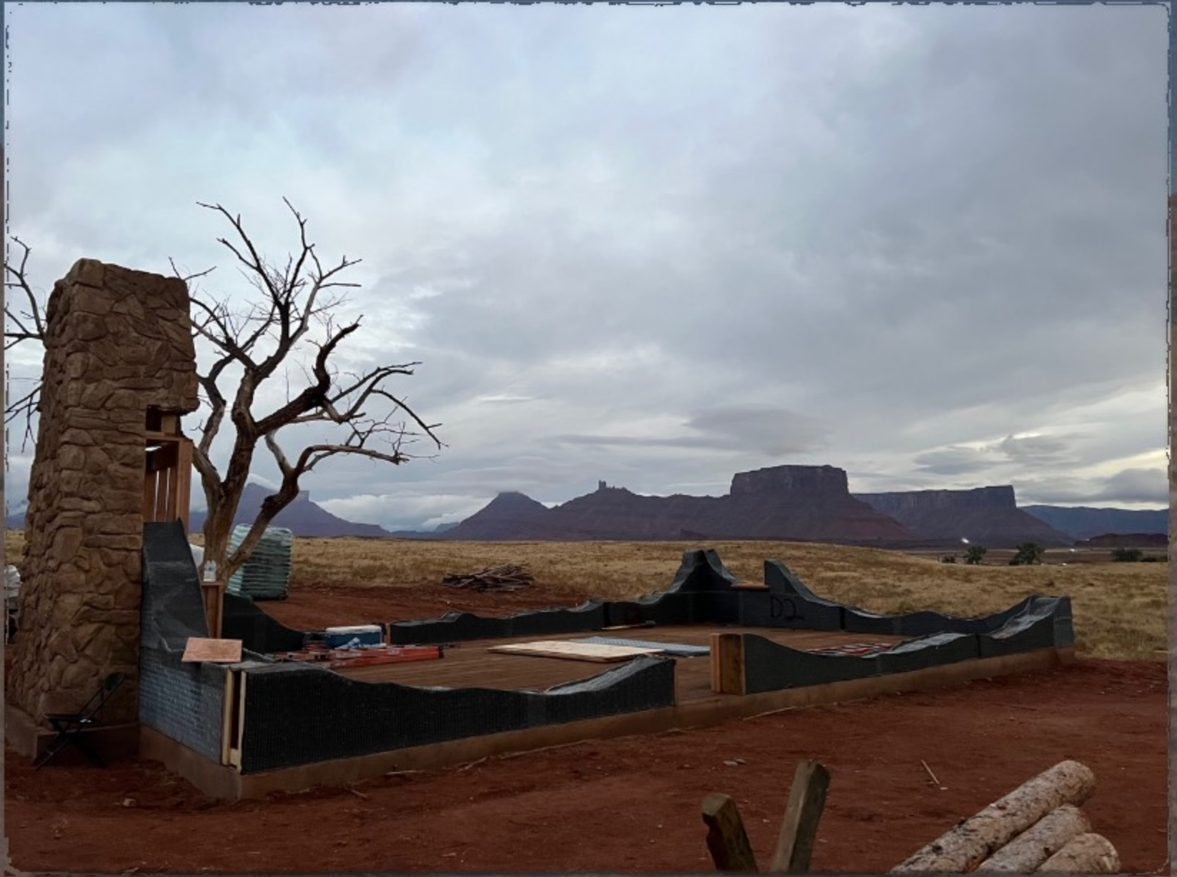
KITTREDGE HOUSE - ON LOCATION BUILD PROGRESS
