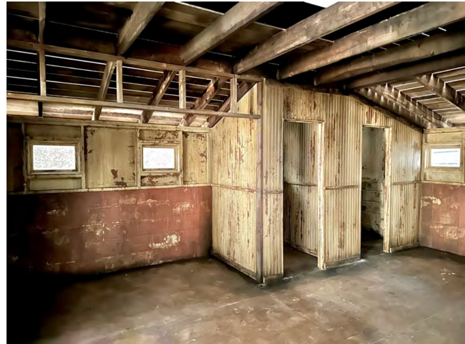
stage set interior construction
