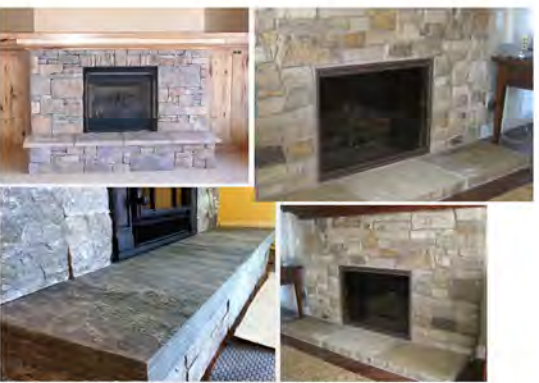
REFERENCE FOR THE GRANITE LIVING ROOM HEARTH. NOTE THE SMOOTH CUT EDGES OF THE BOTTOM LEFT PHOTO
