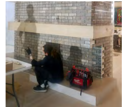
Den fireplace during construction
