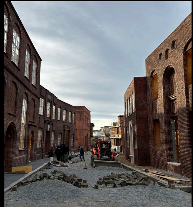
Under Construction - Setting the Grade and Laying Cobblestones
