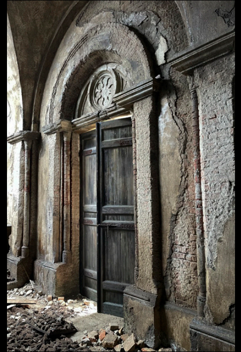
South, Side Door to Chapel - Set Photo
