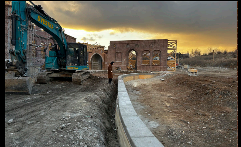
Harding House Exterior Under Construction
