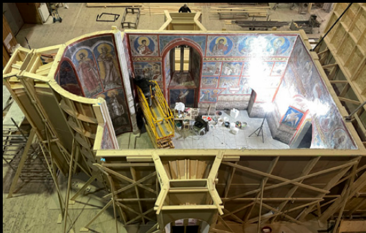
Under Const. (2nd Room - Naos & Apse)
