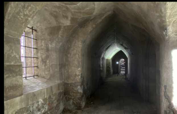
Corridor - Set Photo
