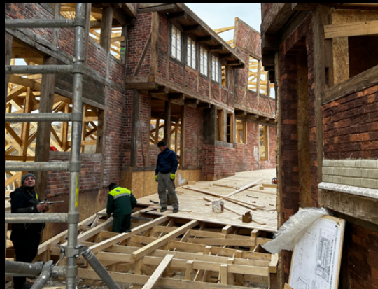
Building the base for Old Town Street
