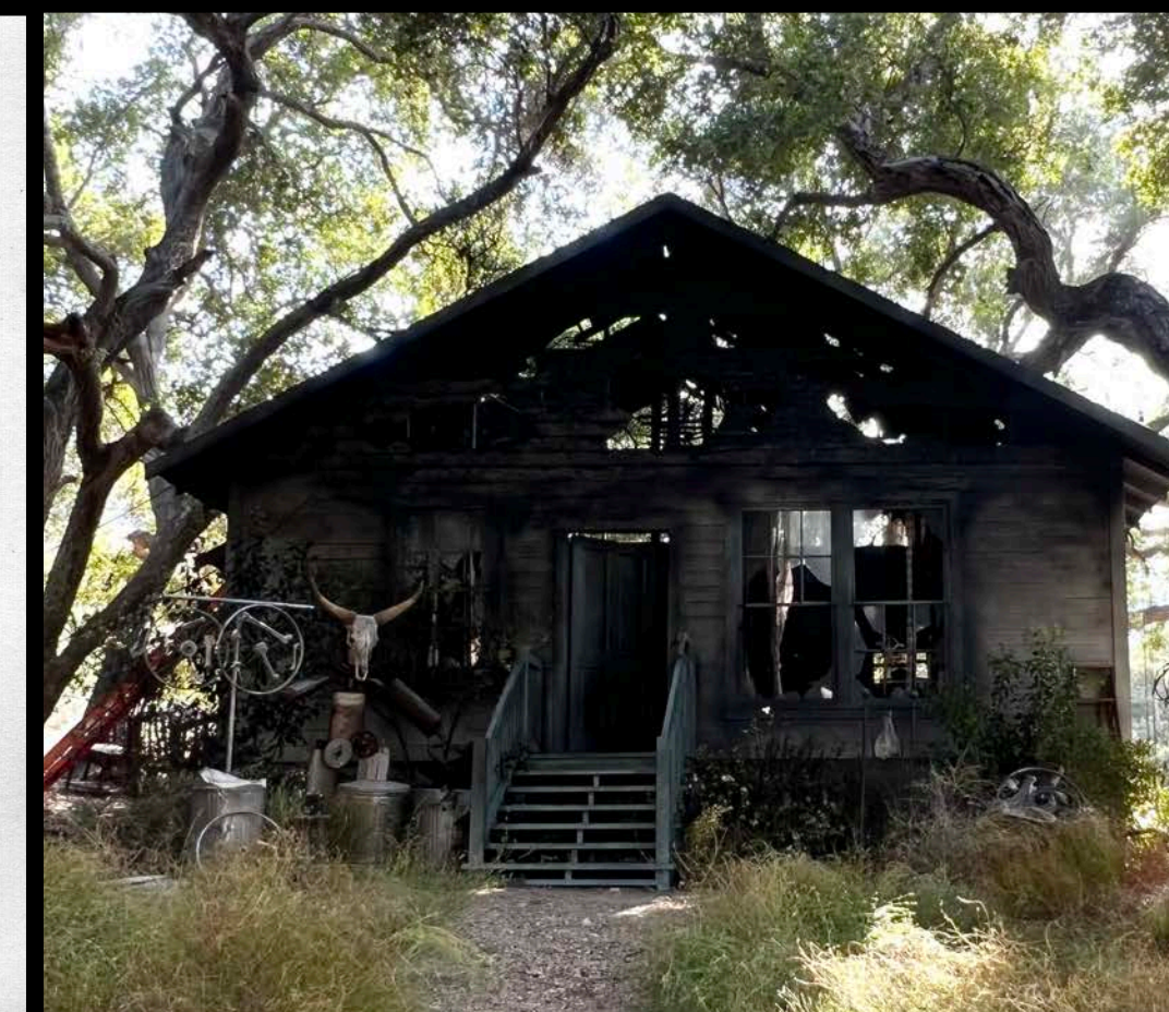
BURNED HOUSE (LOCATION BUILD)
