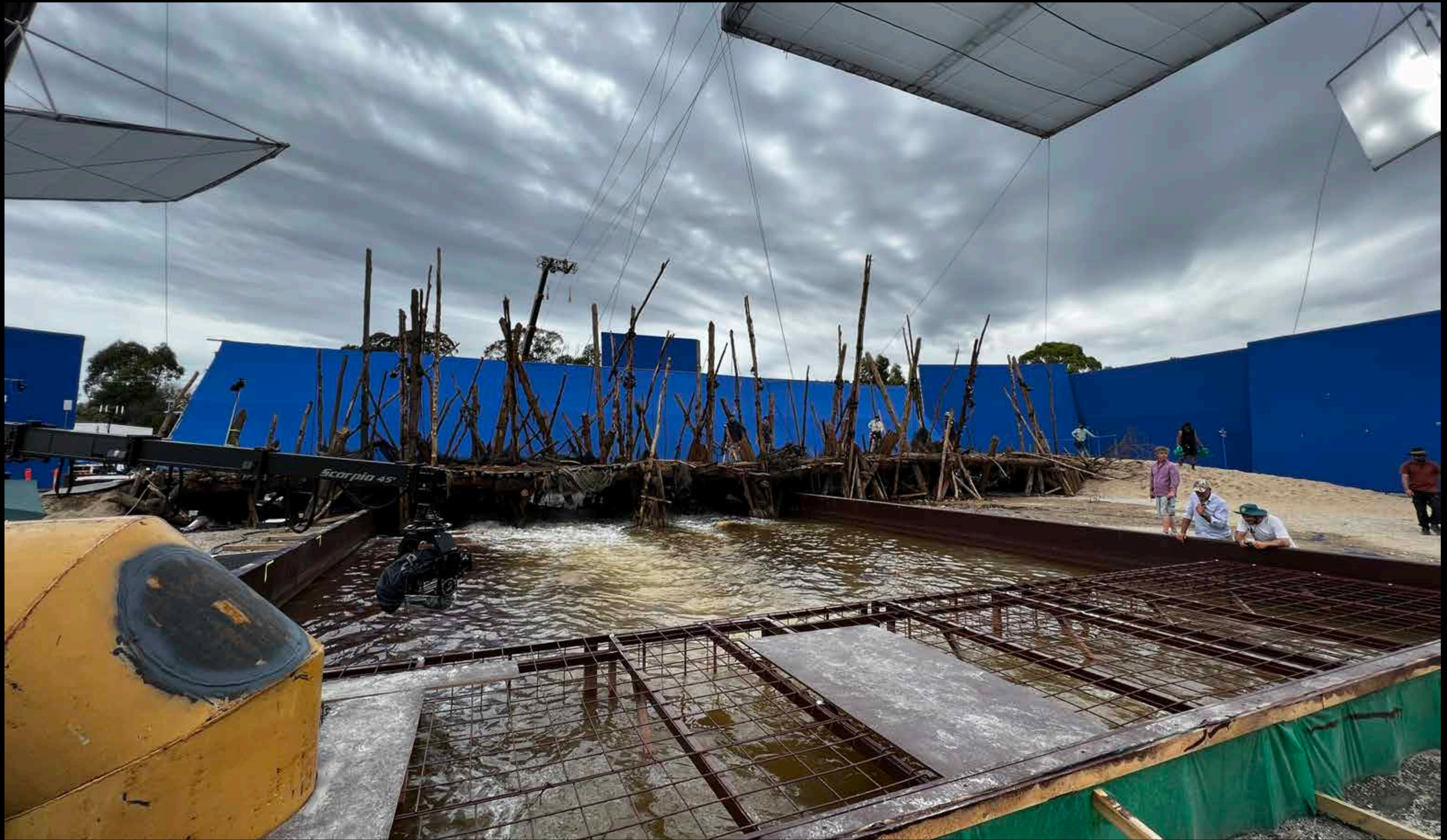
MARAUDERS BRIDGE – BACKLOT BUILD
