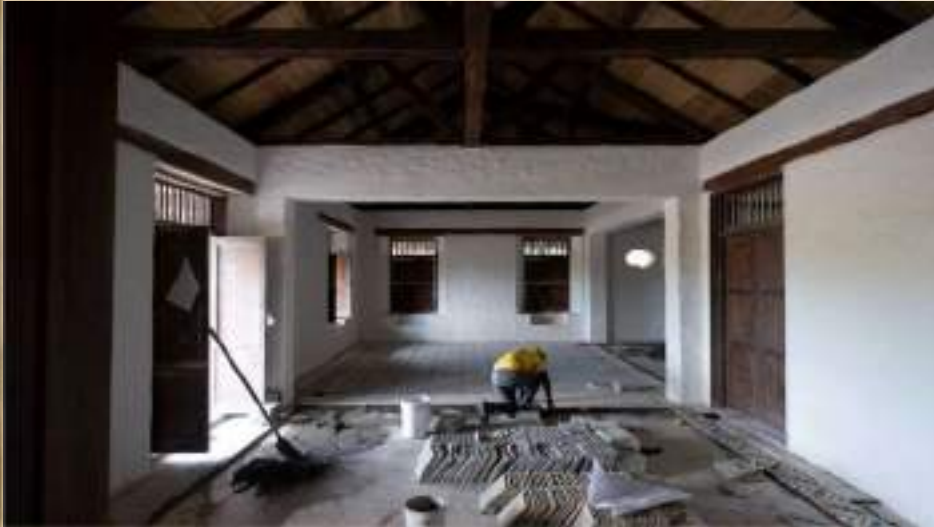
4TH STAGE FLOOR HYDRAULIC TILE INSTALLATION
