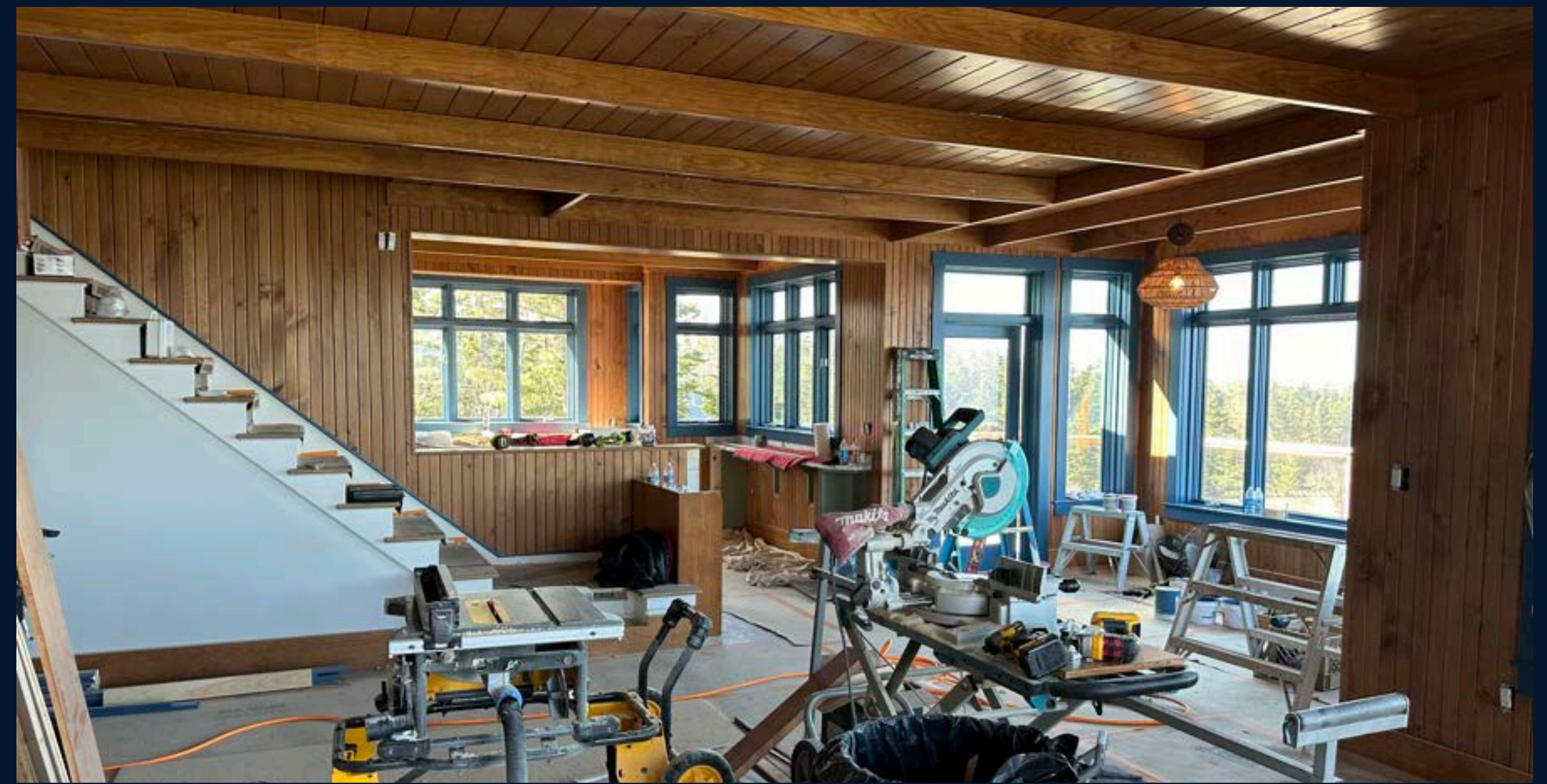
build in progress
