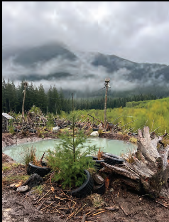
POND BUILD COMPLETED
