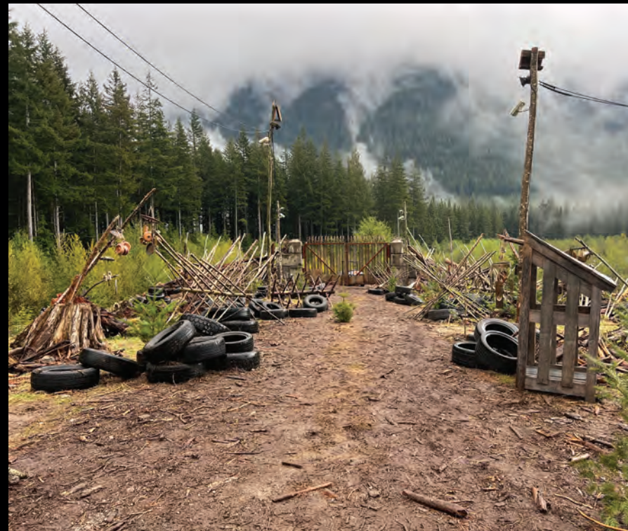
COMPOUND BUILD WIP
