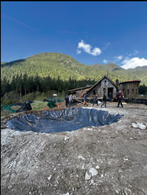
POND BUILD WIP
