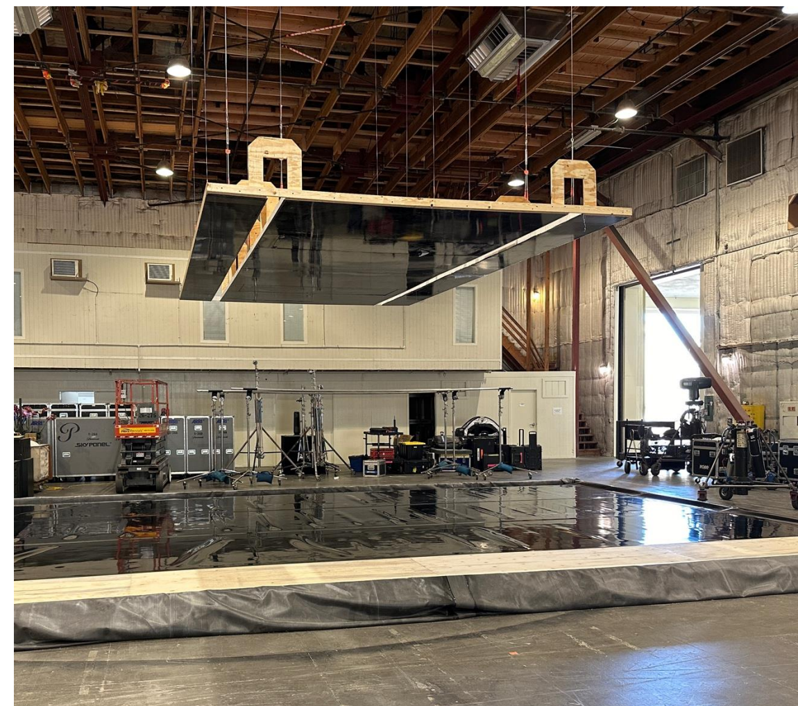
POND LINER UNDER SET FOR RAIN SpFX
